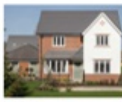
THE ALLOCATED WALK MAY ALLOW FOR A VARIATION IN BACK-TO-BACK DISTANCES WHICH TARGET JOIN AS A BARRIER FOR DEVELOPMENT RESIDENTS & INCORPORATE UP TO JOIN TO ALLOW OPPORTUNITIES FOR A PLANTING STRATEGY TO INCLUDE TREES IN BACK GARDENS.
